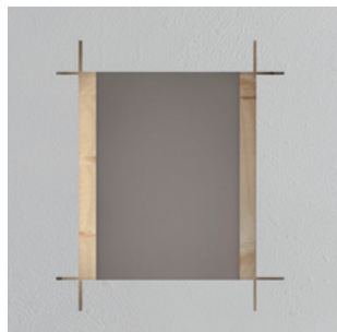
Cut a 222 x 187,5 x 64 mm hole in the wall and install 2 wooden planks
