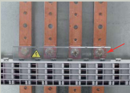
Clip the transparent protective cover on the distribution block
