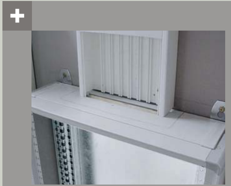
All the enclosures are supplied with an adjustable insulated cable entry plate
