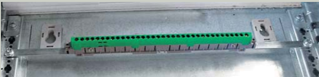
Direct fitting of the flat bar on the functional uprights
