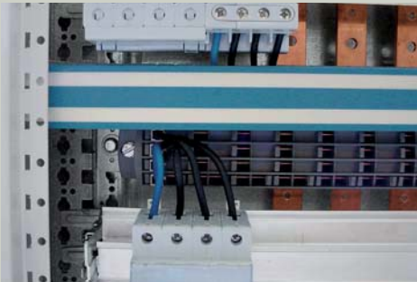
The 75 mm fixing centre enables Lina 25 40 x 60 ducting to be installed for wiring the top row
