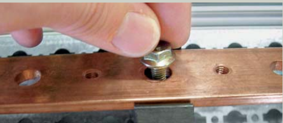
Position the copper bars on the supports
