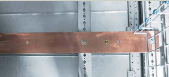
Main terminal consisting of a copper bar at the back of the enclosure
