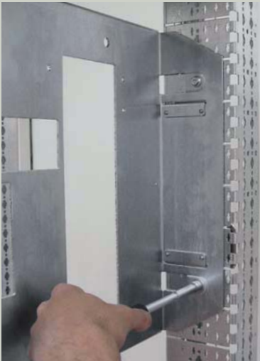
Locking the plate using M6 screws and clip-nuts
