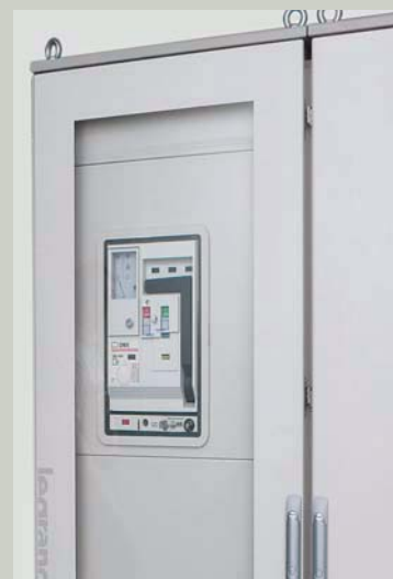
IP 55 protection is obtained by using a door
