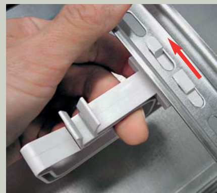
Fitting a guide ring for horizontal wiring
