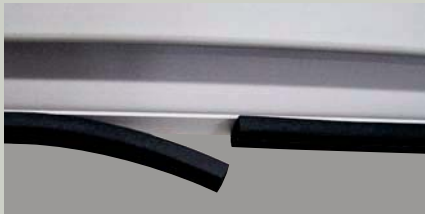
The seal must be fitted in the bottom of the door
