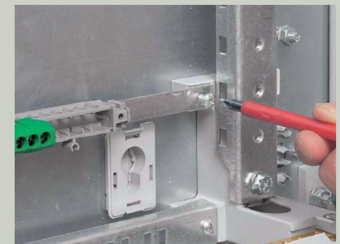
Fix the bar on the plastic supports integrated at the back of the enclosure
