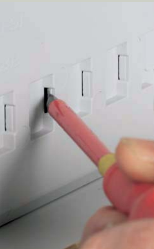
Knocking out the feedthroughs
