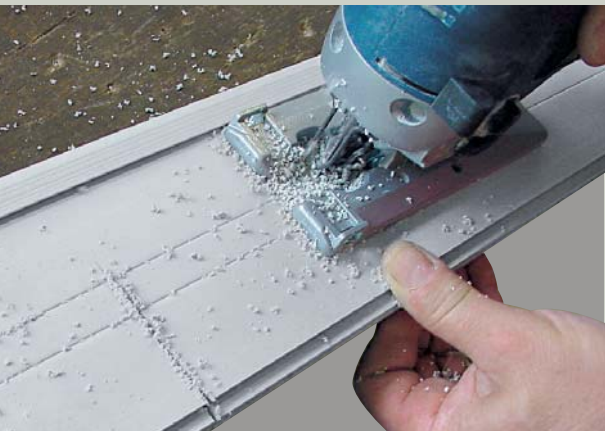
The side panels are easy to cut using a jigsaw
