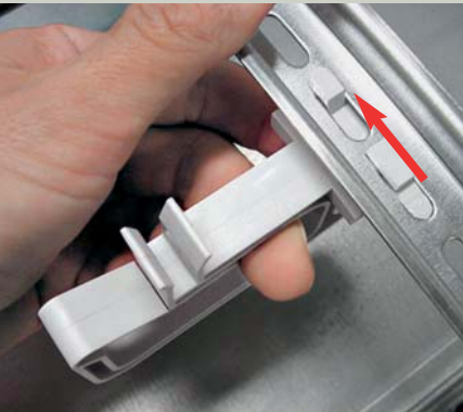
Fitting a guide ring for horizontal wiring
